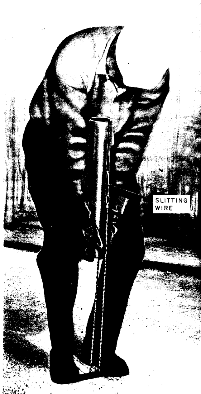
Fig. 2—Using Sleeve Slitter
