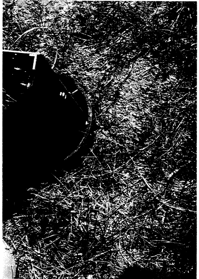
Fig. 4: Fire ant mound infesting pedestal
