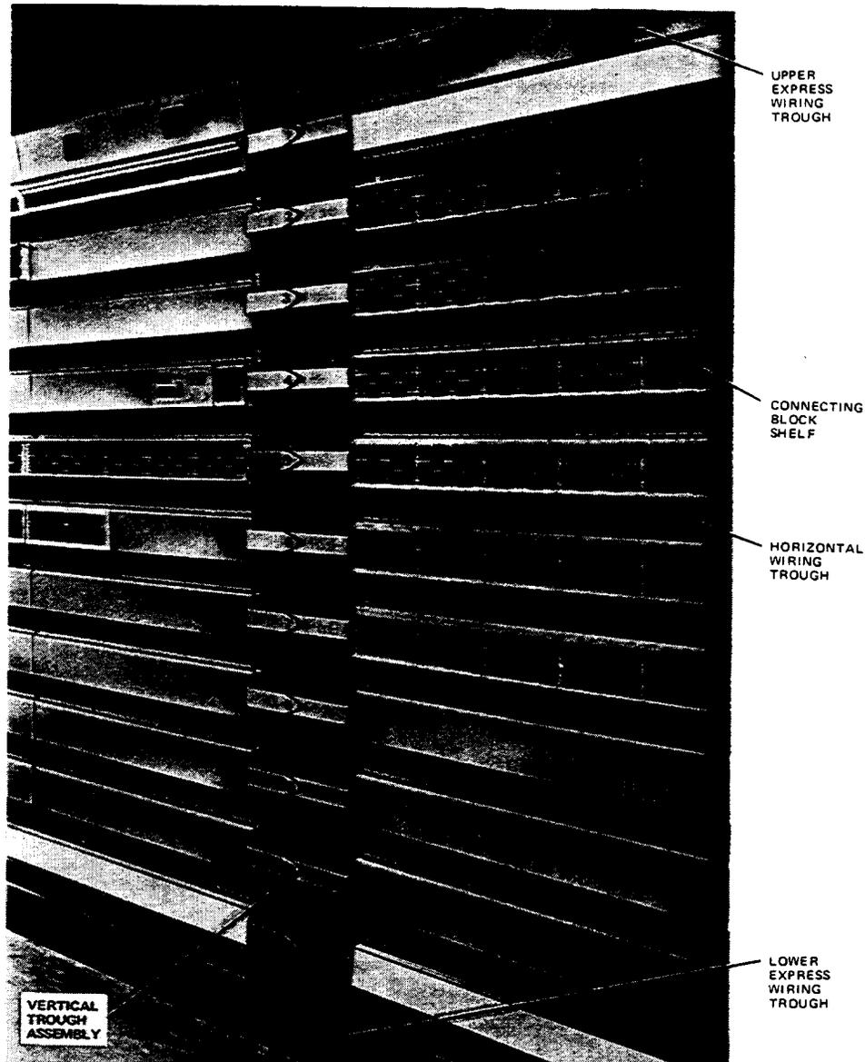
Figure 4—Typical *COSMIC*-Type Distributing Frame (Front View)
