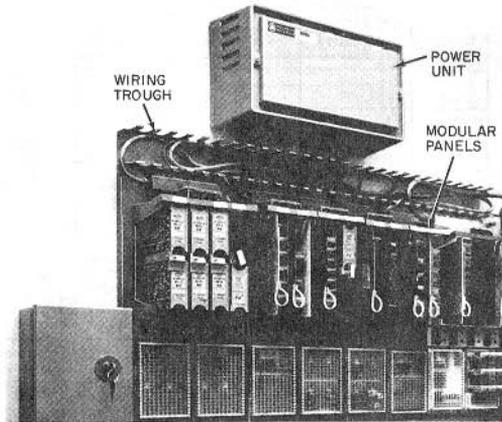
**Fig. 47—Typical Installation of 840348288 Wiring Trough (Cover Removed)**
