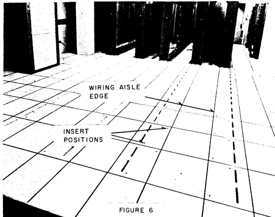
Fig. 6—Support Panel Locations for Fixed Floor Plan and Raised Floor System
