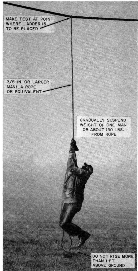
Fig. 2—Testing Strand Prior to Placing Ladder
