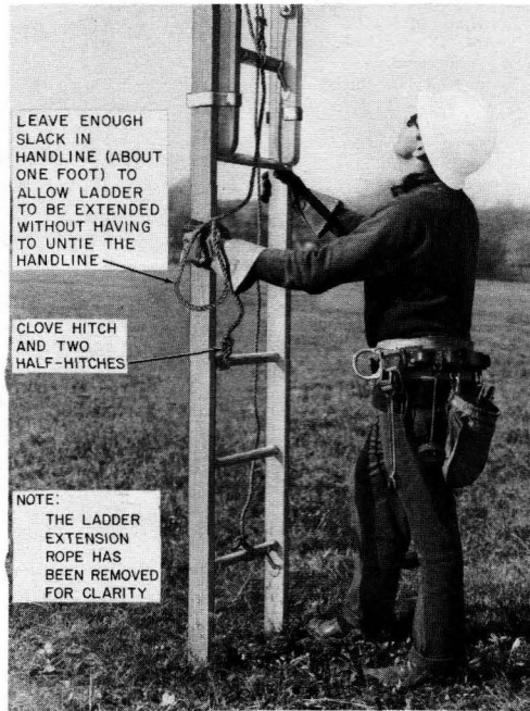
Fig. 20—Method of Securing Handline
