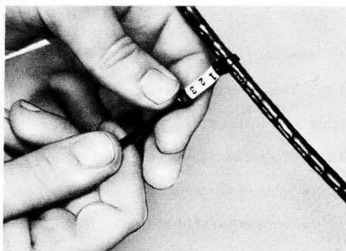
Fig. 2—♦Placing Tie and Marker♦
