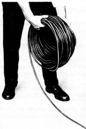
Fig. 2—Paying Out Cable
