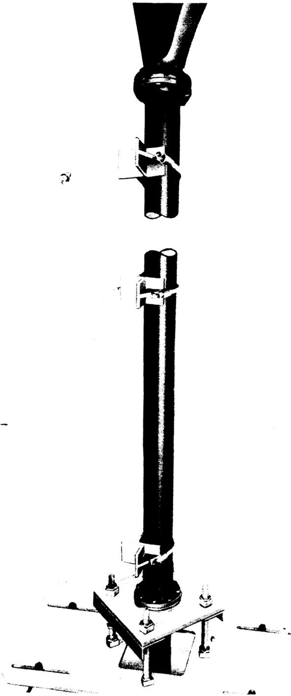
**Fig. 7—Clamps L-501857 Fixed to In-Service Waveguide Before Hanger Plate Lowering**
