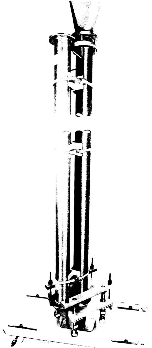
**Fig. 8—Clamps L-501857 as Used to Hold The New Waveguide Section in Place**
