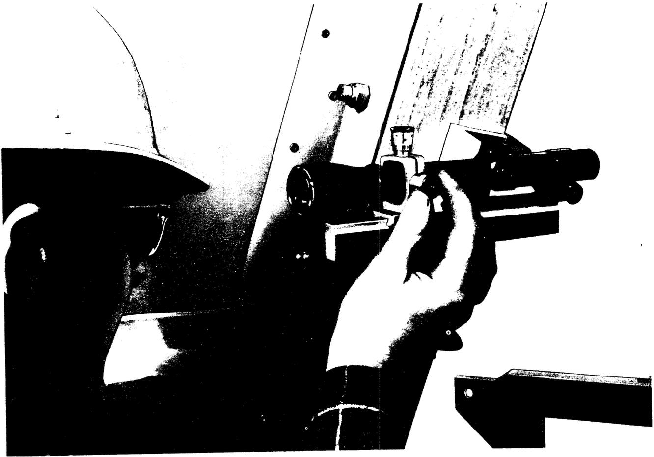
Fig. 13—KS-20073 Telescope Installed on KS-15676 Antenna
