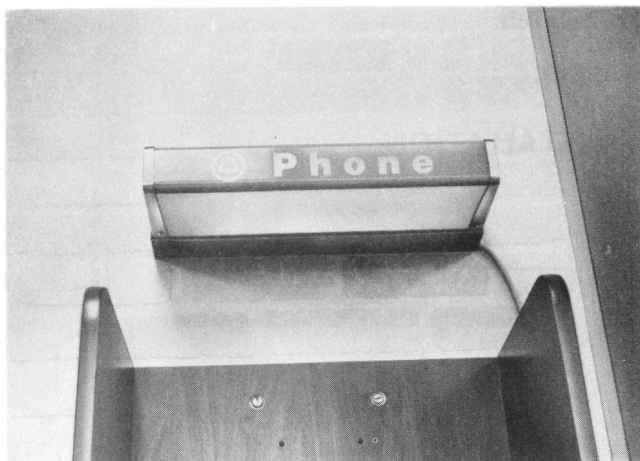
Fig. 4—♦KS-19681, List 9 Sign Installed on List 13 Wall Mounting Bracket♦
