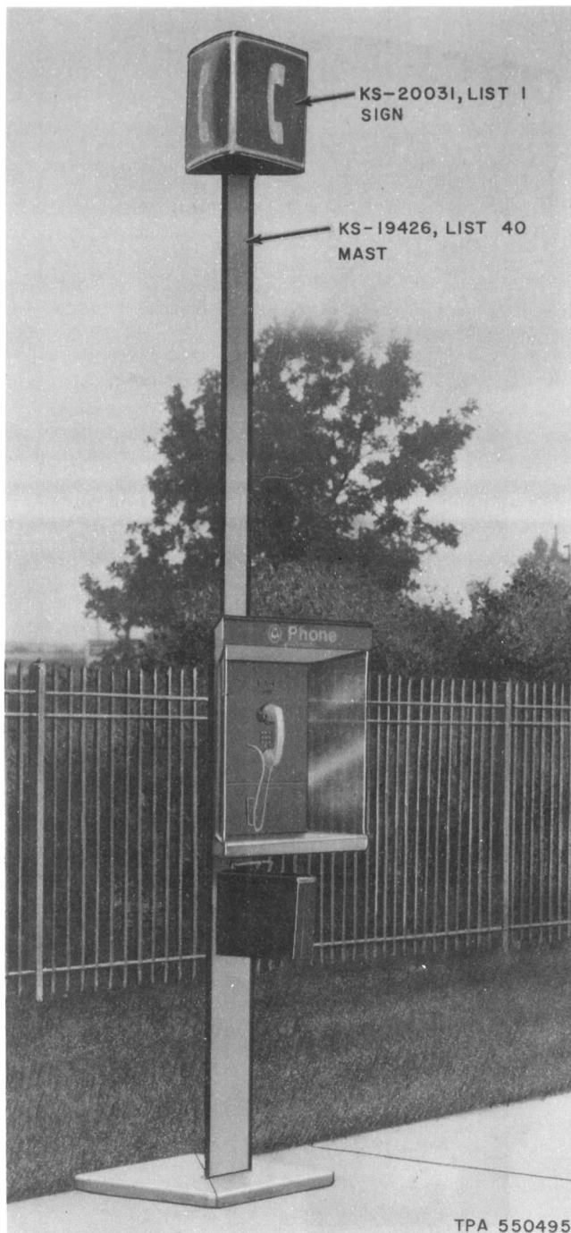
Fig. 23—KS-20031, List 1 Sign Installed on KS-19426 Mounting Without Canopy
