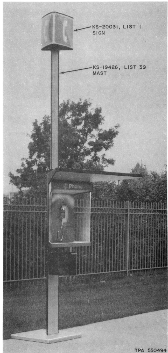
Fig. 22—KS-20031, List 1 Sign Installed on KS-19426 Mounting With Canopy
