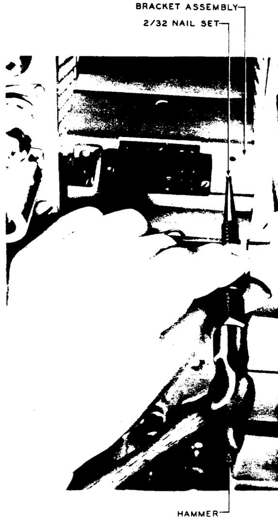
Fig. 5 - Method of Removing Rivet From Bracket
