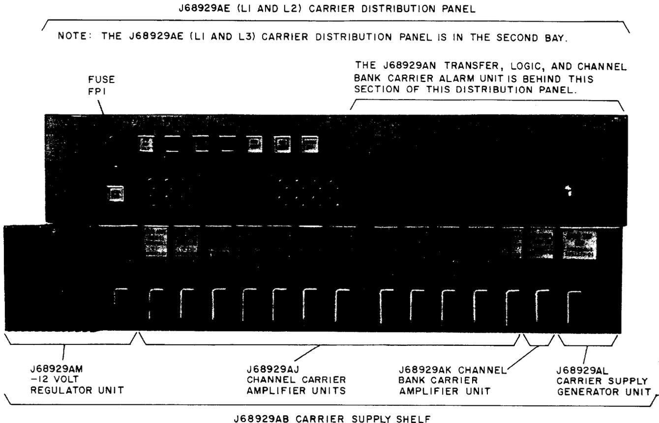
**Fig. 3—A6 Carrier Supply and Distribution Panel**
