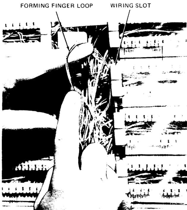
Fig. 6—Forming Finger Loop
