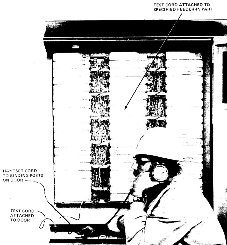
**Fig. 3—Verifying Feeder-In Pair—108-Type Connectors**
