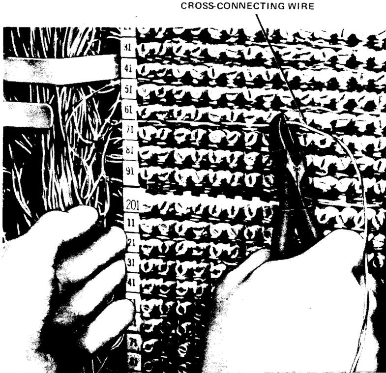
Fig. 12—Cutting Cross-Connecting Wire
