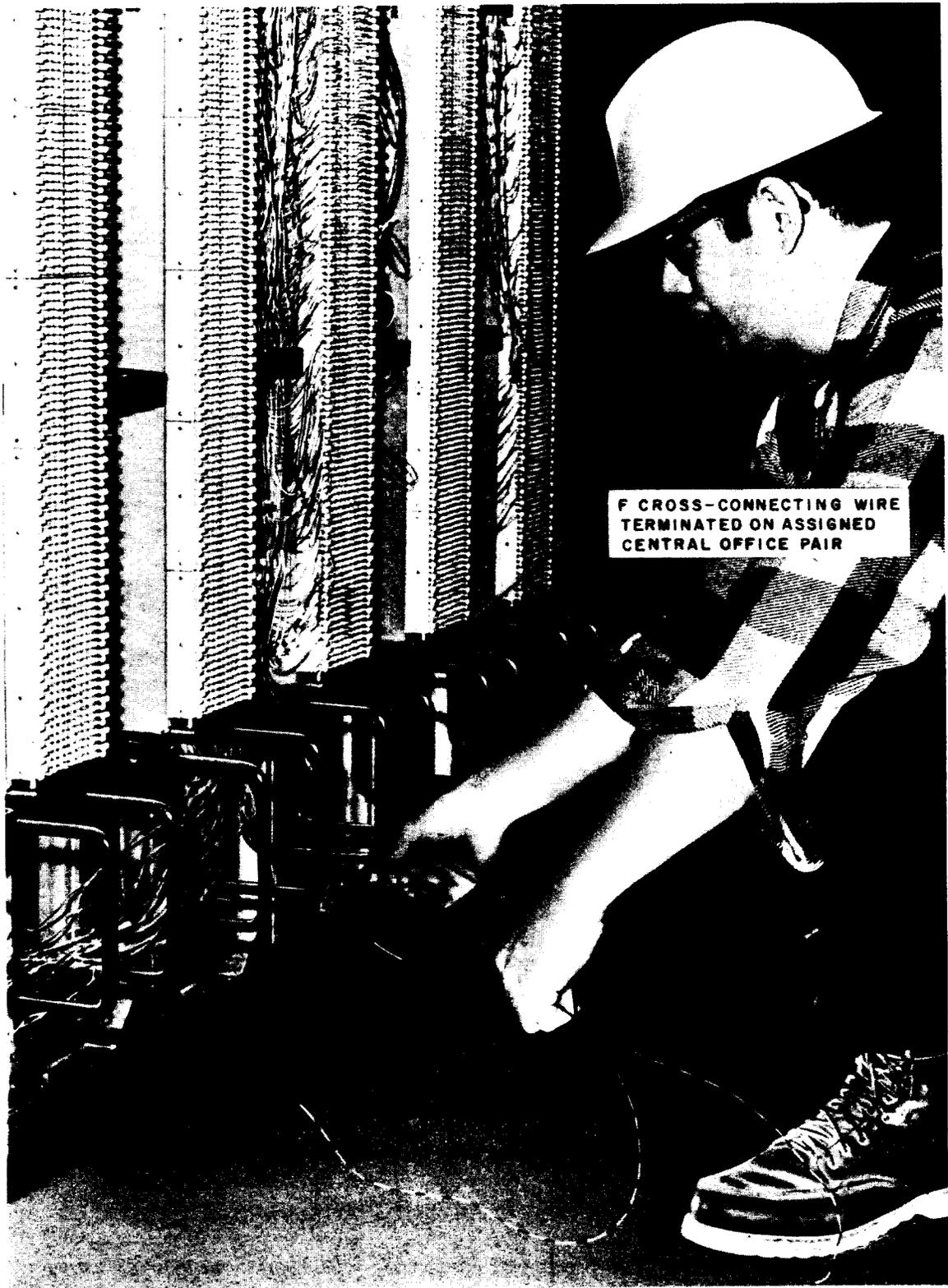
**Fig. 9—Running Cross-Connecting Wire Along The Outside of Bottom Wiring Ring**
