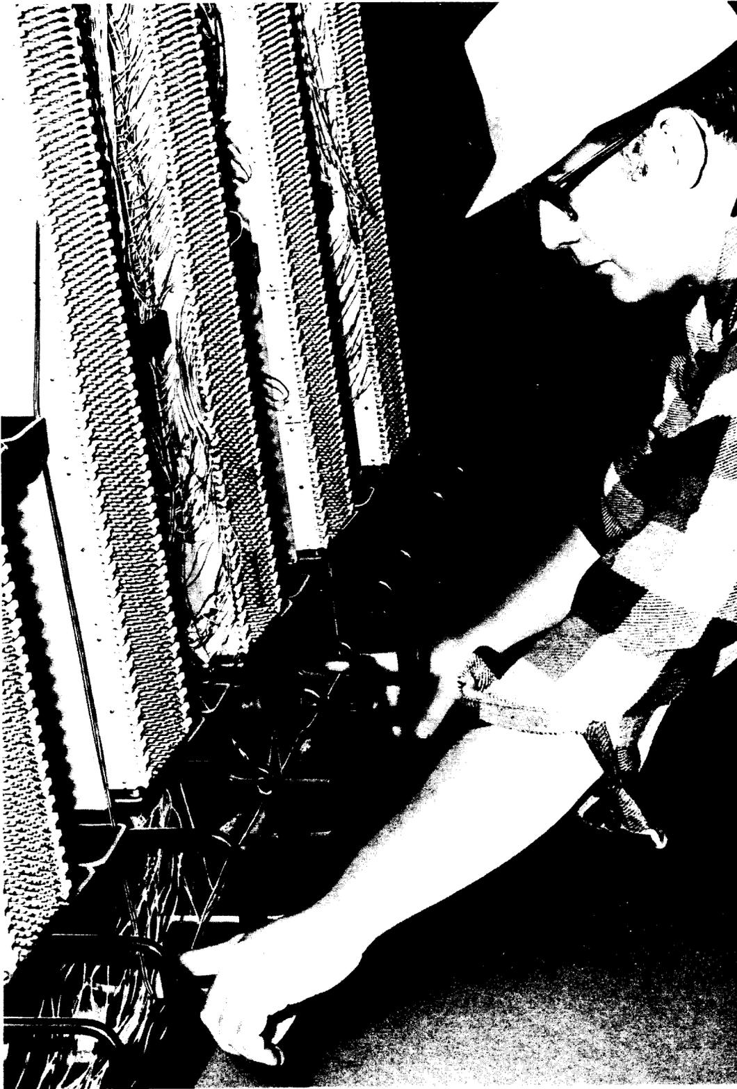
Fig. 12—Positioning F Cross-Connecting Wire in Bottom Wiring Ring
