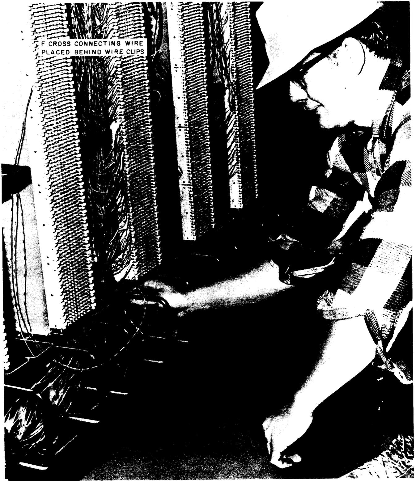
Fig. 11—Placing F Cross-Connecting Wire in Bottom Wiring Rings
