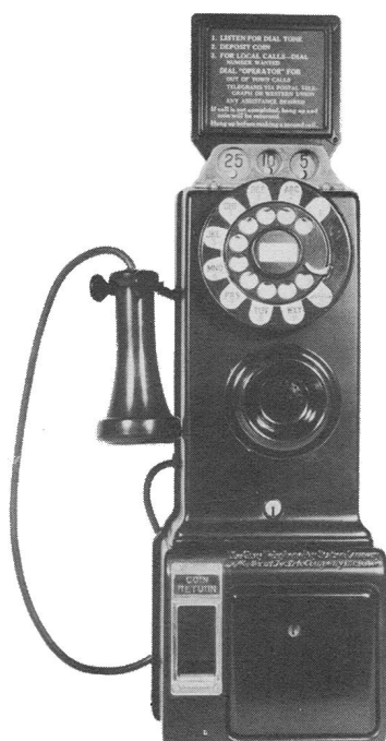
Wall Telephone for use in dial exchanges Dimensions: Width 9" Depth 8 \frac{3}{4} " Height 22 \frac{7}{32} "
