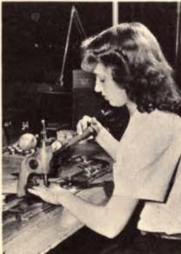
Performing an assembly operation in the manufacture of the transmitter for the "500" set. The operator is fastening a gold-plated electrode to the transmitter diaphragm. The operation is a precise one, because the parts must nest together in order to meet the close tolerances required.
