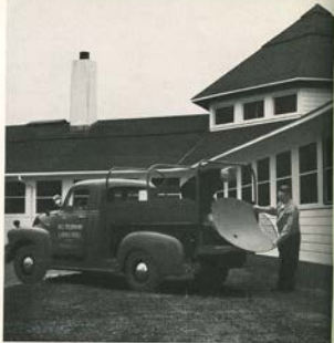
Fred Luth (left), Holmdel's only motor pool driver, and John Warneker of Service Staff unload antenna dish at main building.
