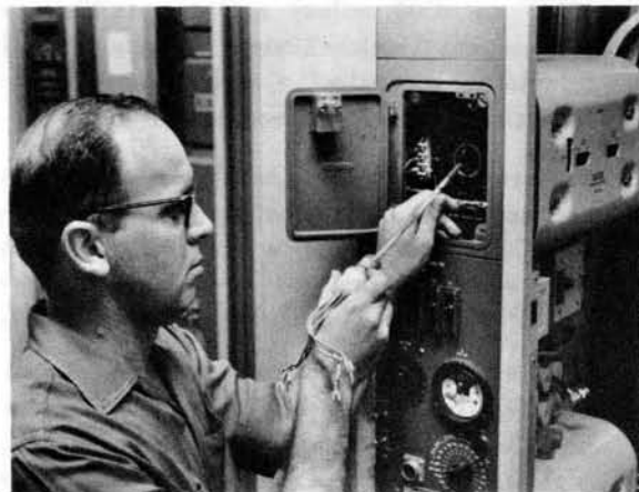
INSTALLER REPLACING TRAVELING WAVE TUBE
