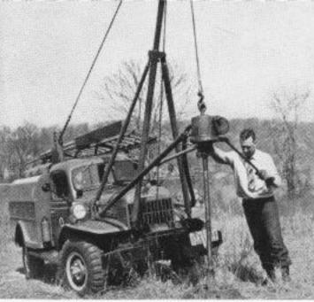
Power driven augers, as pictured above, help speed the construction of rural telephone lines. At left: Linemen string wires to serve more farm telephones.
