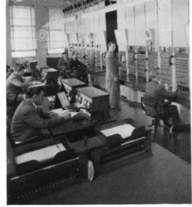
Long Lines control board and equipment for setting up radio broadcasting networks for transmission of programs over telephone circuits.
