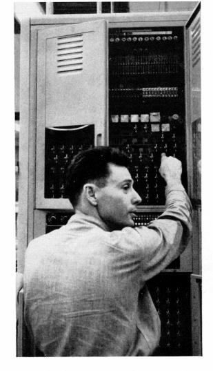
Above W.E installer L. R. Bayse tests circuits associated with the AMA computer in new Washington installation of centralized automatic message accounting. Installers have long since left. Their handiwork remains as shown in overall view (below) of the equipment room containing the new CAMA equipment.
