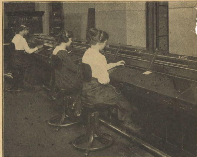
Figure 19. Typical installation of Cordless B positions
