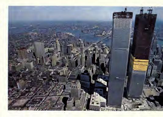
of rentable space. When completed, it will have required 200,000 tons of Japanese steel, 600,000 square feet of tempered, heat-reflective glass and 5,000 construction workers on the site at one time. It will take a 49,000-ton system of air conditioning to cool the place.
