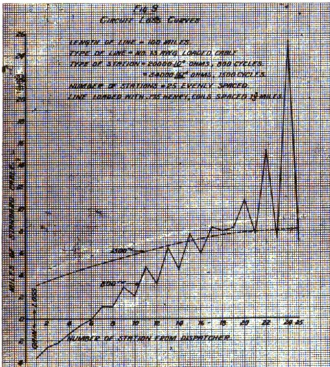
Fig. 9—Curve of Losses on a 100-Mile Line
