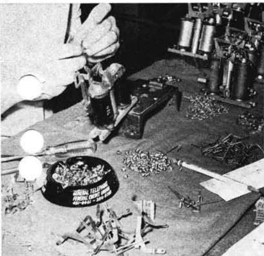
Fig. 4 Reassembling two-coil prepay coin control relay.
